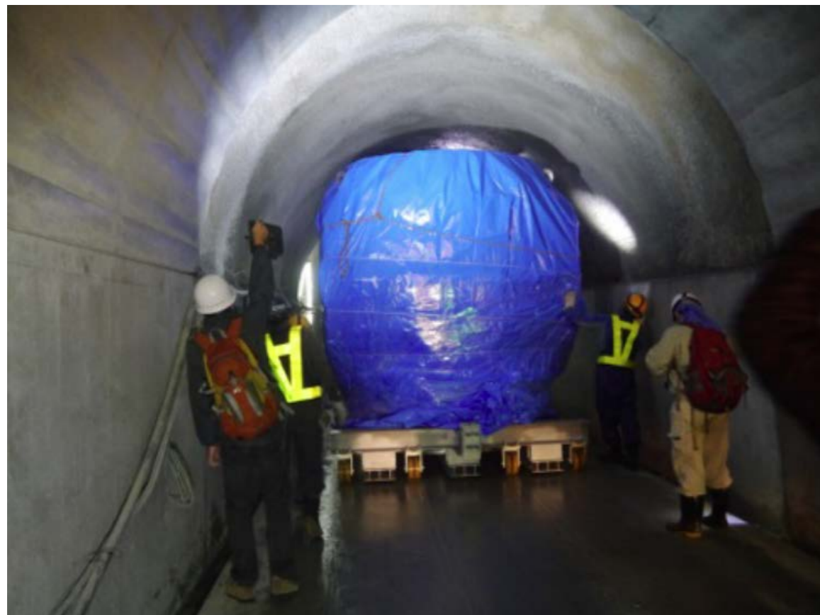
Transportation of cryostat in Y arm
