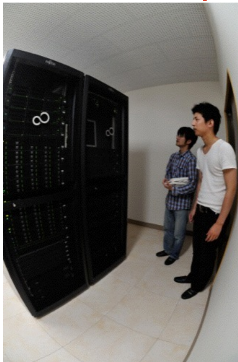
placed at computer area beside the control room, 1st floor of analysis build.
